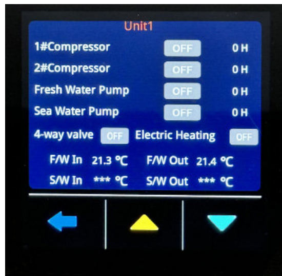
Status screen 2 – outputs and water temperatures
